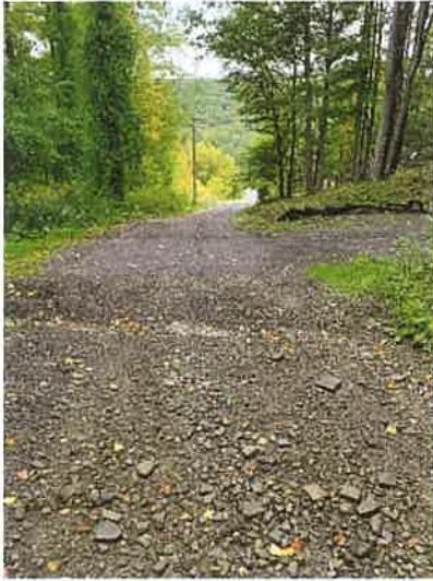
Photo 6 north perspective of service road
